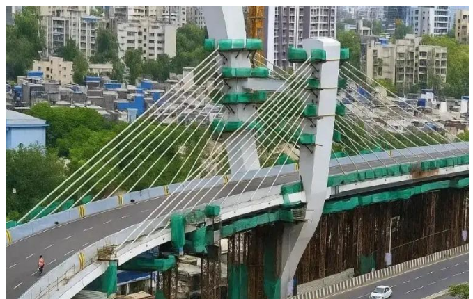
Exhibit 27 : Santacruz-Chembur Link Road's cable-stayed bridge
